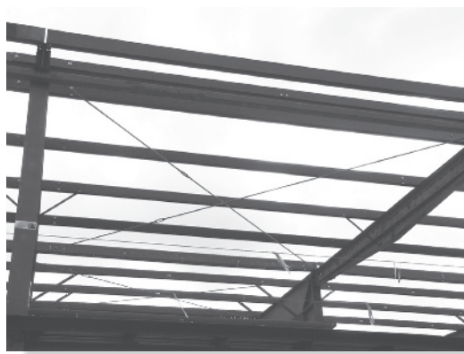
Tie rods are used for cross bracing to stiffen the roof of a building to resist wind loads.
